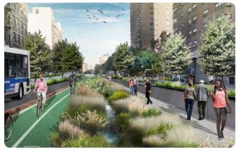
One of the team's proposed pilot projects to combat the bathtub effect in East Harlem was an integrated stormwater management/green infrastructure project along 106th Street paired with a reconfiguration of the right-of-way to better accommodate pedestrians, cyclists, and buses.
